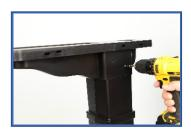
Attach Bracket (part B) to the top of the Mailbox Post (part C) as shown using (4) #12x 1" Self Tapping Screws (part E). There are 4 pre-drilled holes in the bracket. Screws will go into the post with slight pressure. Do not over tighten.
